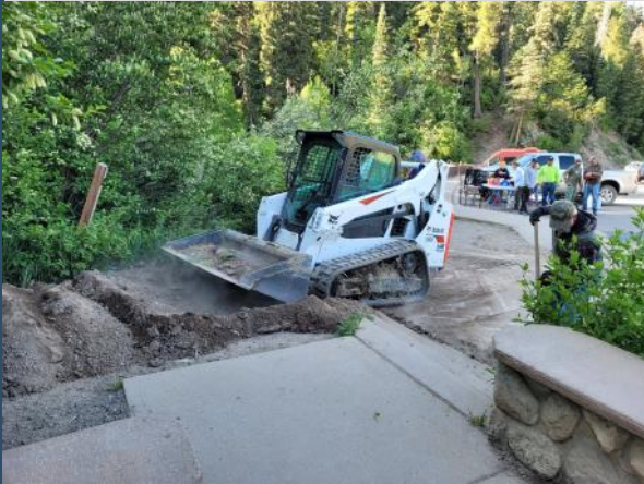
At left—Randy Betts saved the group hours of work by using his skid steer to remove compacted dirt and gravel that washed down the trail. At right—Workers (from left) Steve Earle, Randy Senzig, John Nelson, Ron Toland and Rob Lambert construct one of two rolling dips on the trail to minimize future erosion.
