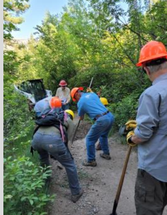
At left—Randy Betts saved the group hours of work by using his skid steer to remove compacted dirt and gravel that washed down the trail. At right—Workers (from left) Steve Earle, Randy Senzig, John Nelson, Ron Toland and Rob Lambert construct one of two rolling dips on the trail to minimize future erosion.
